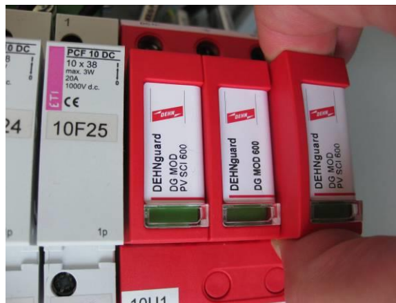
Figure 5.3 Removing of a damaged surge arrester
