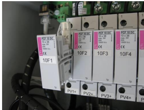
Figure 5.1 Fuse link opened
