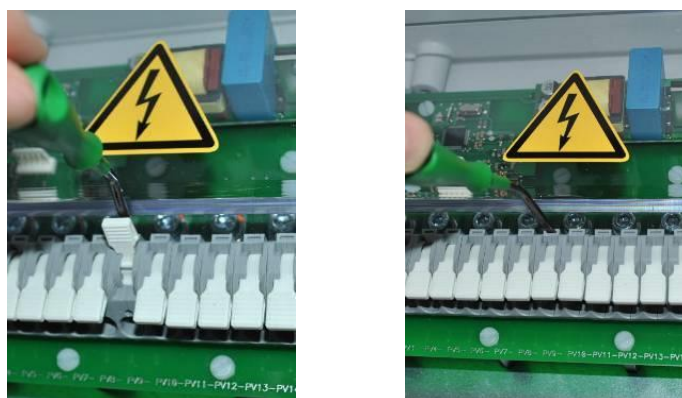
Figure 3.15 Closing a clamping spring-cage terminal for PV(-) string connection without fuse protection
