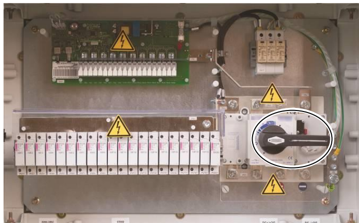
Figure 3.6 Manual switch of the SSB-P
