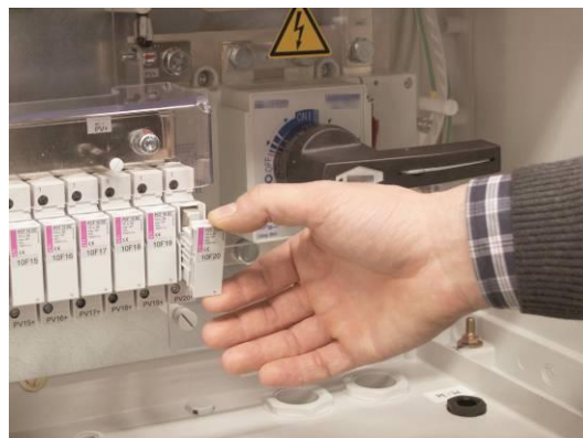
Figure 5.1 Fuse link opened
