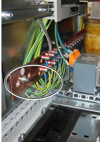
Figure 4.13 PE – copper rail (see also Figure 4.9-2)
