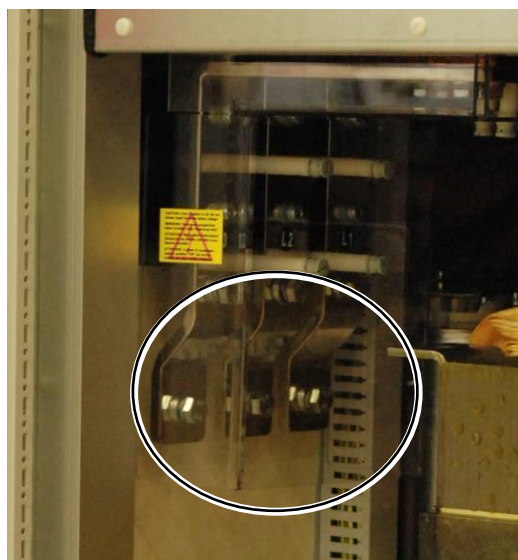
Figure 4.12 Phase terminals (see also Figure 4.9-3)
